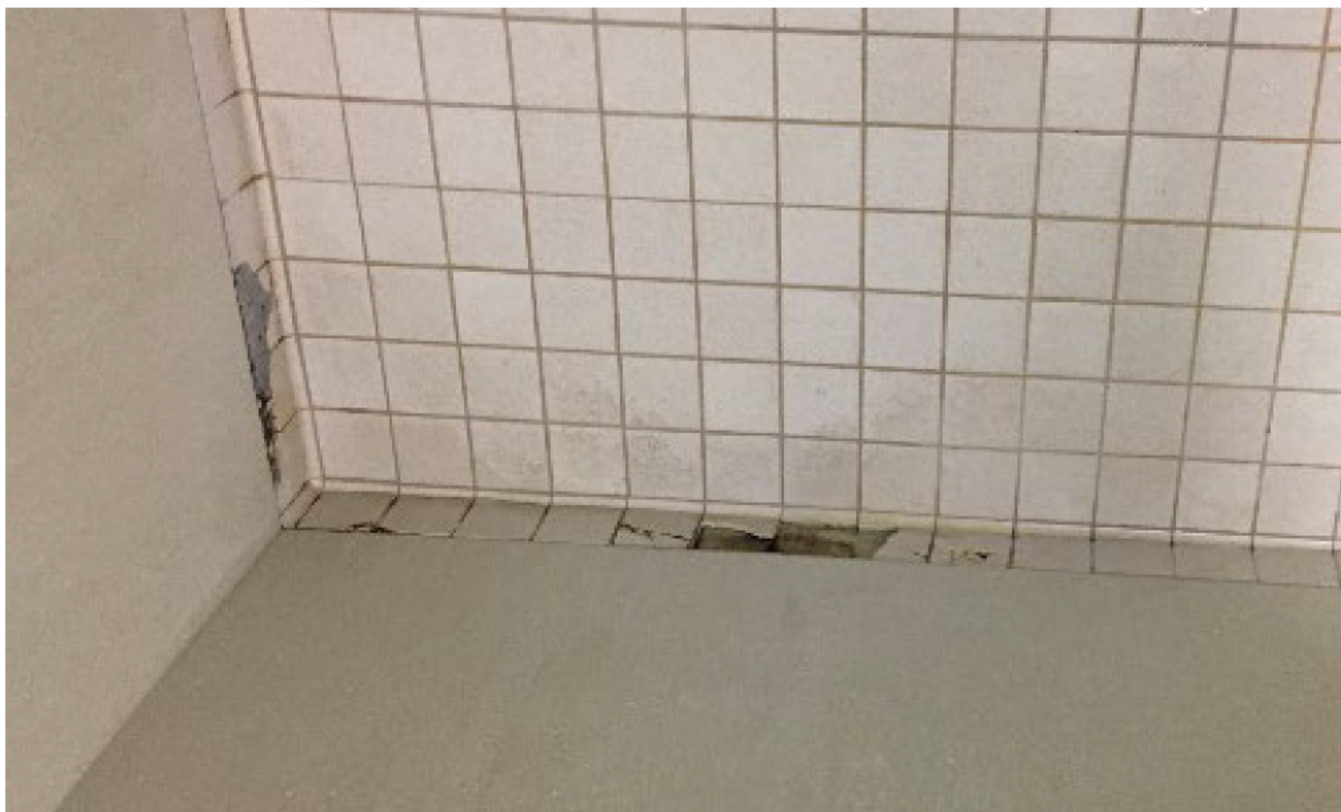
Above and Below: Two examples of the deteriorating infrastructure. These photos are from the bathroom/shower areas of one of the living units. Tiles are cracked and missing.
